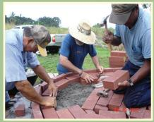
also installed. A rock and cement trough was built in the front to accommodate the coals that are dragged out of the oven before the bread is baked. The oven was left to dry for about a month and the rebar was taken out. In January 2006, a volunteer came faithfully every other
