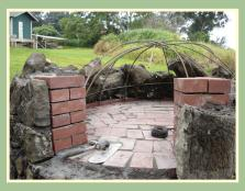
day for 2 weeks to "cure" the oven. At first he built small fires for 15 minutes then gradually worked up to several hours, so that the stones and cement would heat slowly to avoid cracking.
